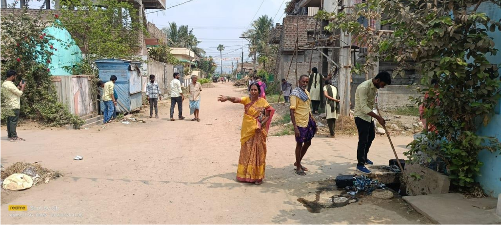
NSS Volunteers clearing garbage in drains
